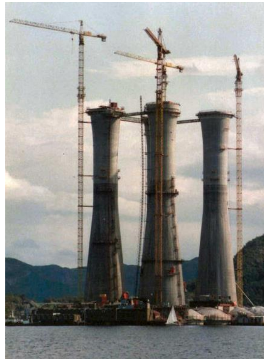
Figure 19.3 – Tapered Slip-forming 19.1
