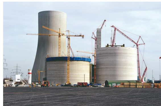
Figure 19.4 – Slip-forming of Fuel Tanks 19.2
